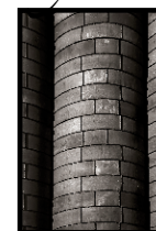
Cole Thompson The Art of Grain Silos
